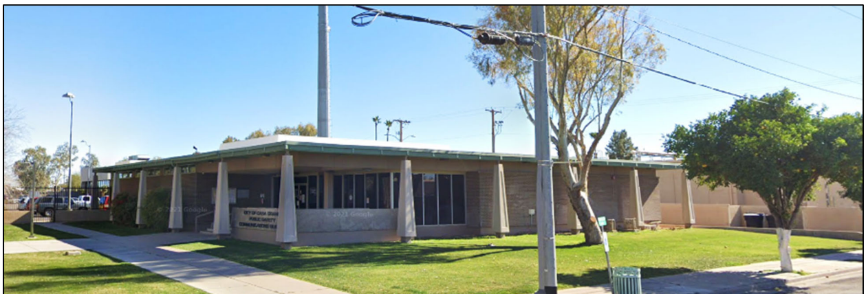
Figure 88. Cit Hall Annex (Department of Public Safety) (LS 103) at 520 N Marshall Street.
